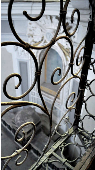
FIGURE 15 The view on the chancel through the grating. PHOTO: AUTHOR.
